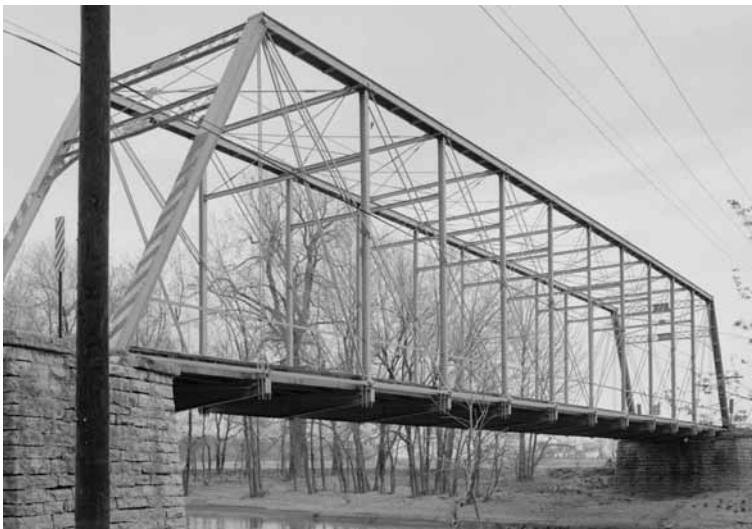
9. Wabash River Bridge, State Rt. 316, Wells County, IN
