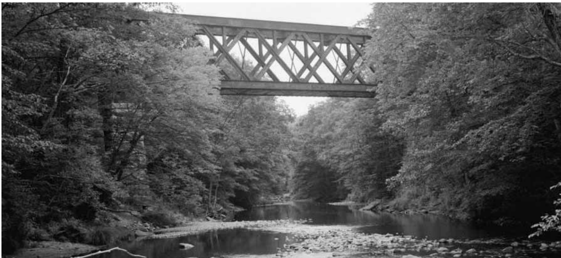
18. Bridge over Blackledge River, Colchester, New London County, CT
