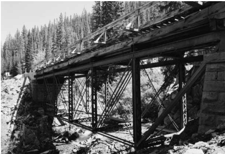
7. Denver South Park & Pacific Railroad Bridge, Romley, CO
