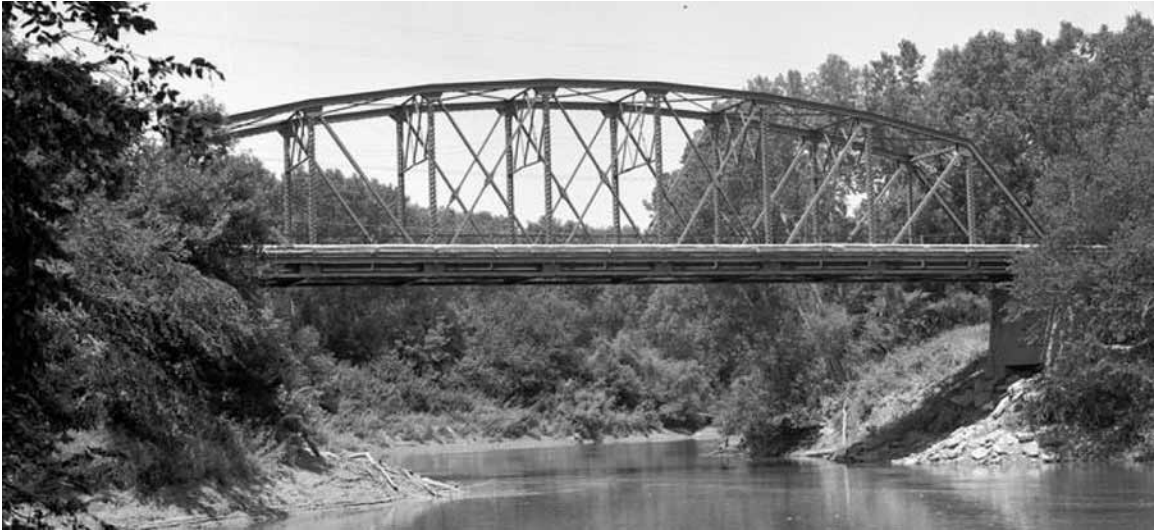
19. Enterprise Bridge over Smoky Hill River, Highway K-43, Enterprise, Dickinson County, KS
