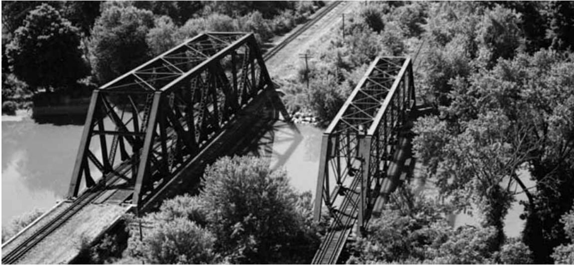
16. Baltimore & Ohio Railroad Bridges, Cattaraugus County, NY
