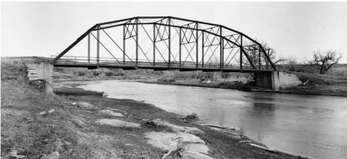
15. Arvada Bridge over Power River, County Rd. No. 38, Sheridan County, WY
