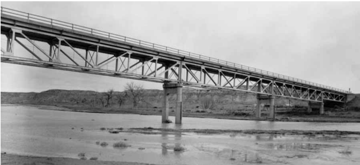
26. Powder River Bridge, Arvada, Sheridan County, WY
