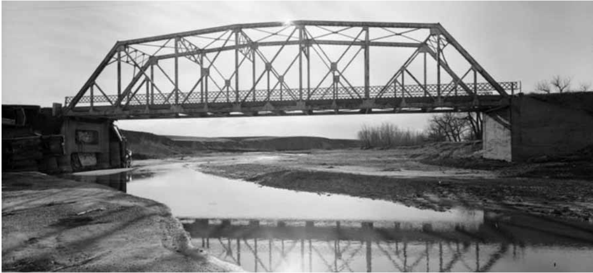
10. Cheyenne River Bridge, County Rd. 46, Niobrara County, WY
