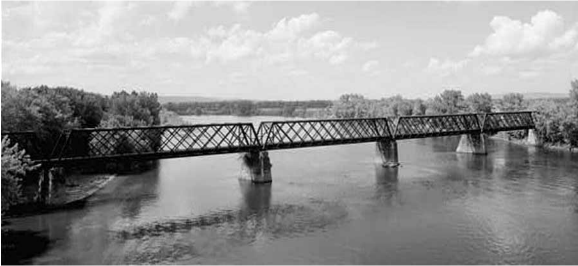
13. Boston & Maine Railroad Bridge over Connecticut River, Northampton, MA
