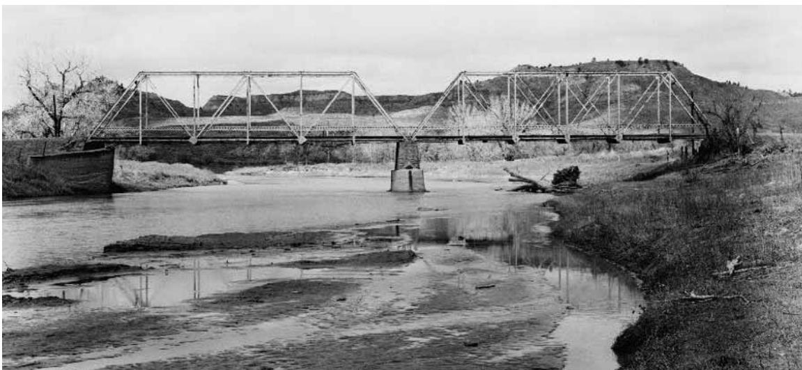
24. Powder River Bridge, County Rd. 269, Sheridan County, WY
