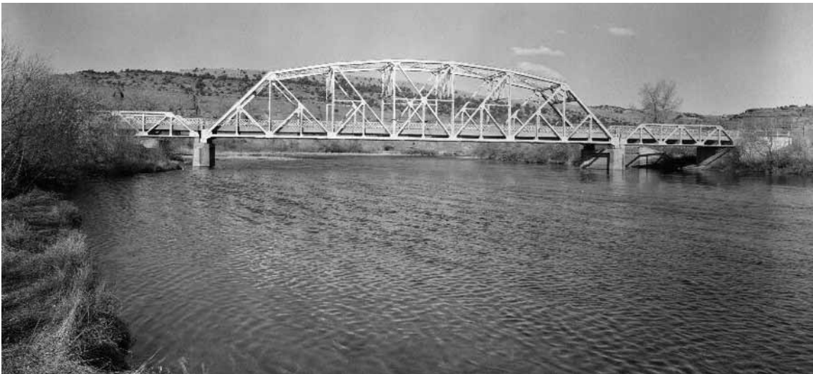
20. Four Mile Bridge over Big Horn River, County Road No. 173, Hot Springs County, WY
