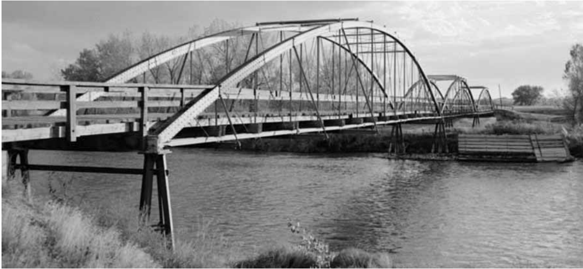
22. North Platte River Bridge, Fort Laramie, Goshen County, WY
