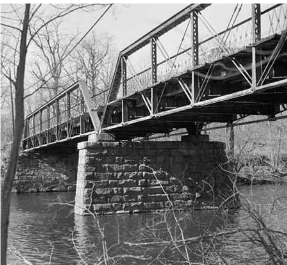
3. Albion Bridge over Blackstone River, Cumberland, RI
