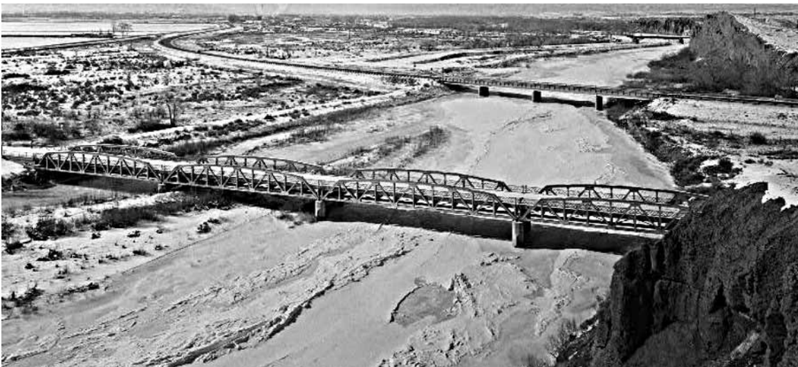
27. Shoshone River Bridge, County Road 111, Big Horn County, WY
